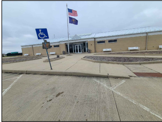
1. View of Centerville westbound rest area south exterior facing north.
